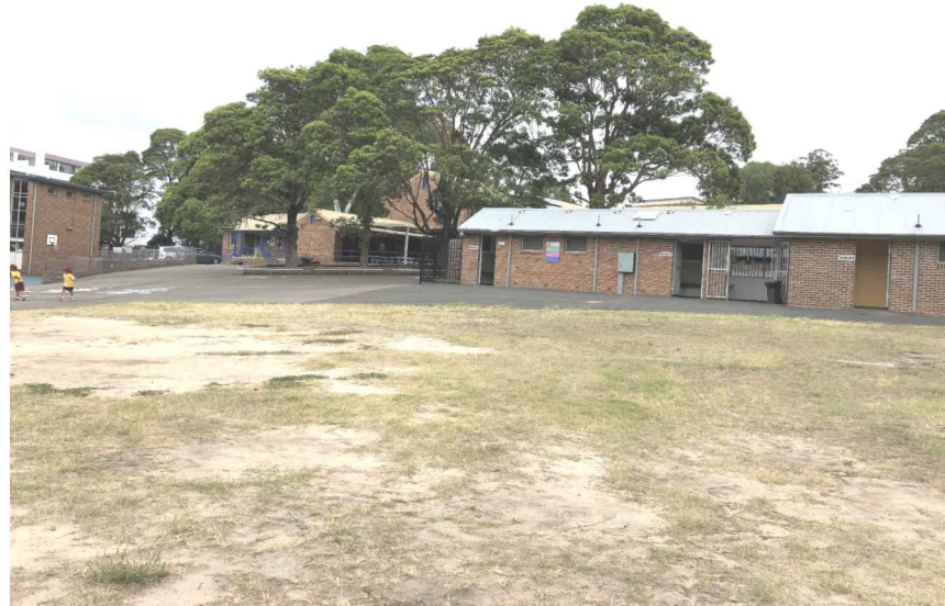
SITE PHOTO - P 2
