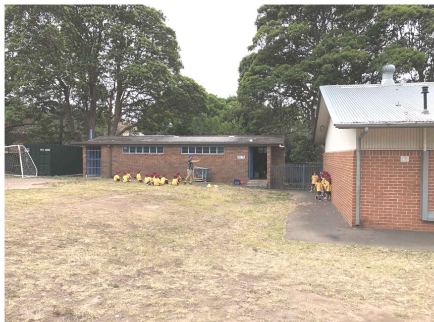
SITE PHOTO - P 3
